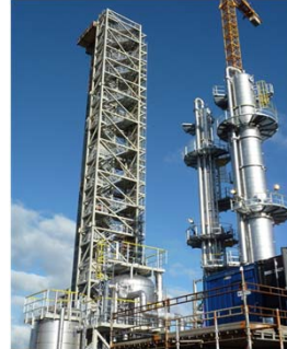
Technology Centre Mongstad, absorber and desorbers
