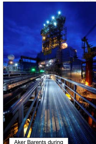
Aker Barents during completion at Stord
